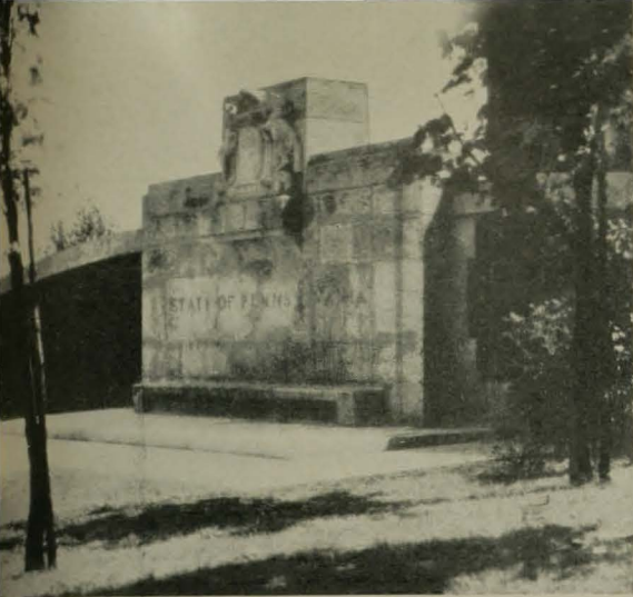
Fountain in Nantillois Erected by State of Pennsylvania
