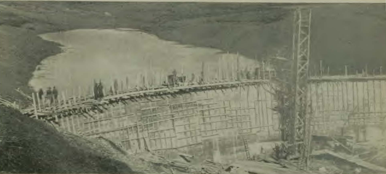
Storage Dam at Savenay Being Constructed by American Engineers
