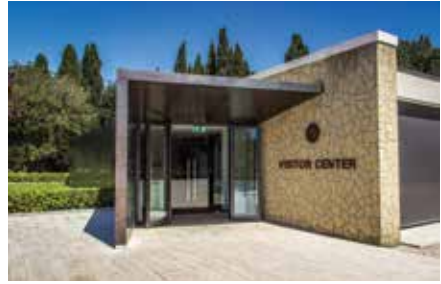
Entrance to the Visitor Center. (ABMC Photo/Richard Arsenault)
